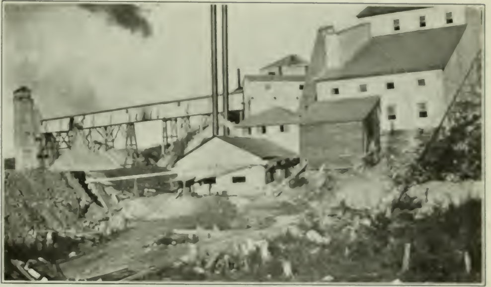
McKinley-Darragh shaft house and mill, Cobalt.
